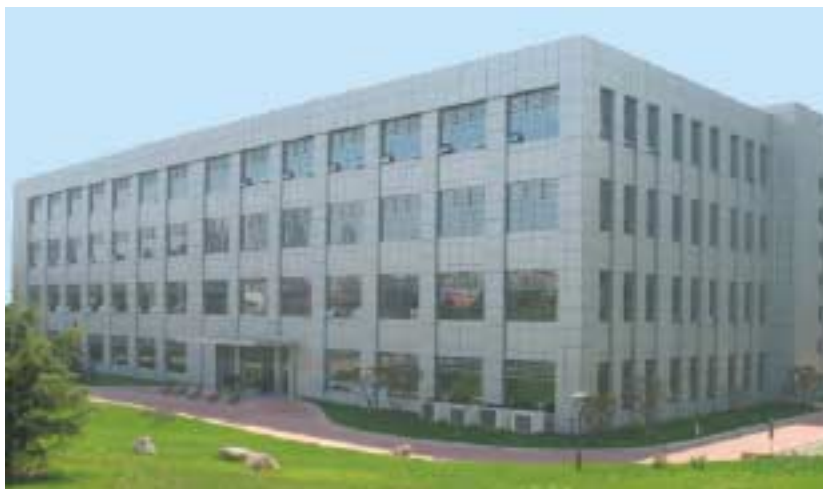
Ligent Photonics Manufacturing Facility Qingdao, China
